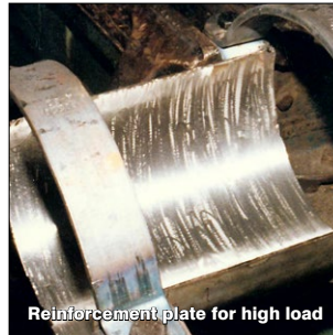
Pipe repair under field conditions
